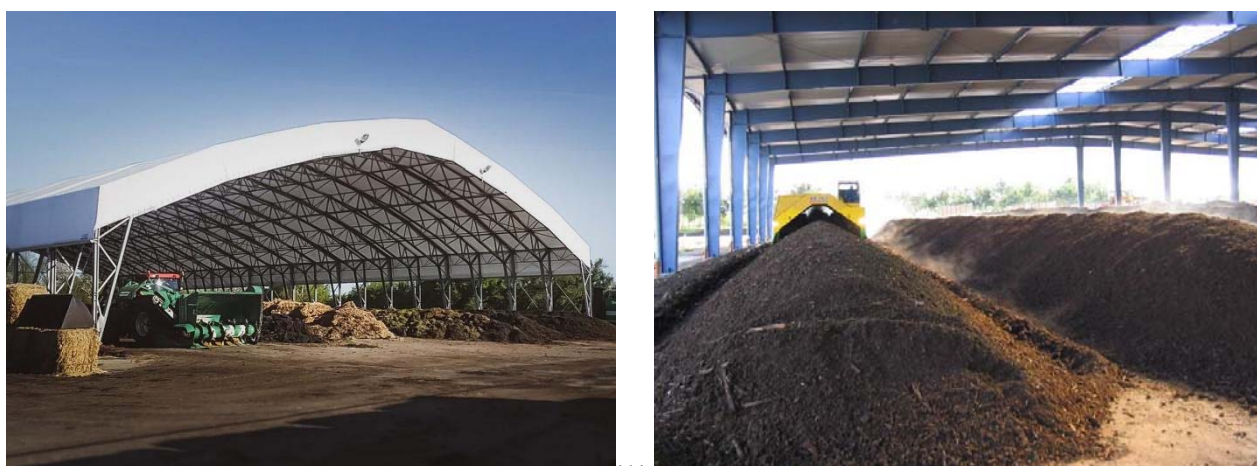
Figure 1.13 – External view of the composting facility in clamps under the roof (source: https://www.compost-systems.com/en/solutions/sheltered-windrow-composting and https://tehnix.hr/en/ )
